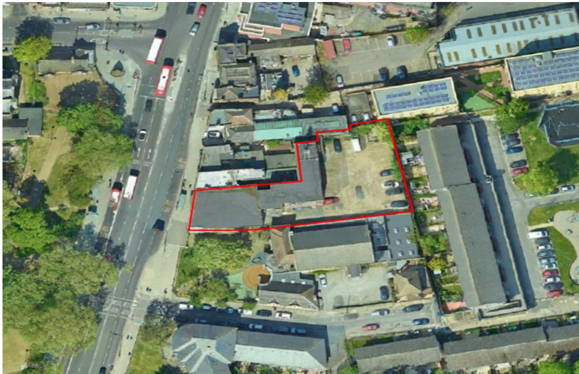
Aerial view of the site and surroundings
