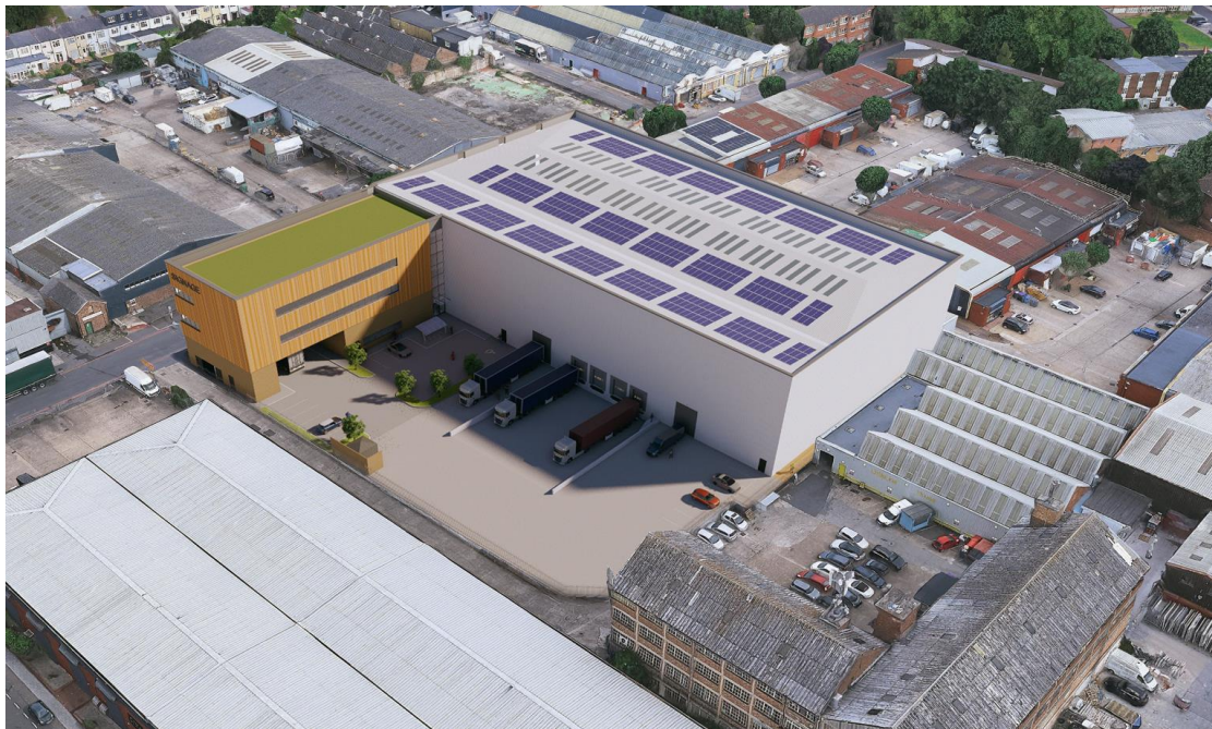
Image 7: Rear of building showing service yard
